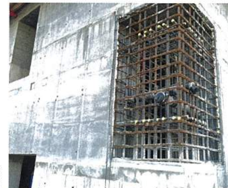
↑ FIGURE 11: 'Leave-outs' at corners of core for outrigger construction
